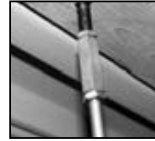
Figure 4: Threaded Rod Assembly
